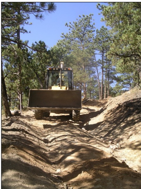
PHOTO: WILDLANDS RESTORATION VOLUNTEERS
